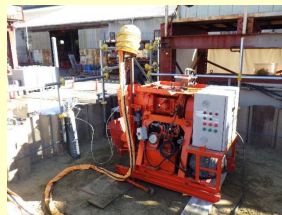
Chemical grouting method (boring and grouting)
