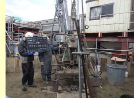
Standard penetration test (SPT)
