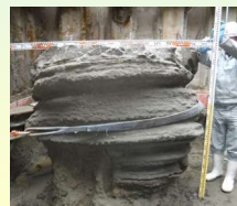
Measuring grouted soil
