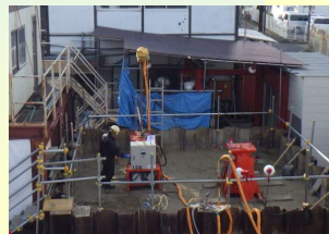
Chemical grouting method (boring and grouting)
